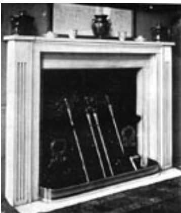
Even the fireplace of the Drawing Room in Soane's House is strikingly vacant of the projecting shelf that is the minimal version of the classical entablature.
