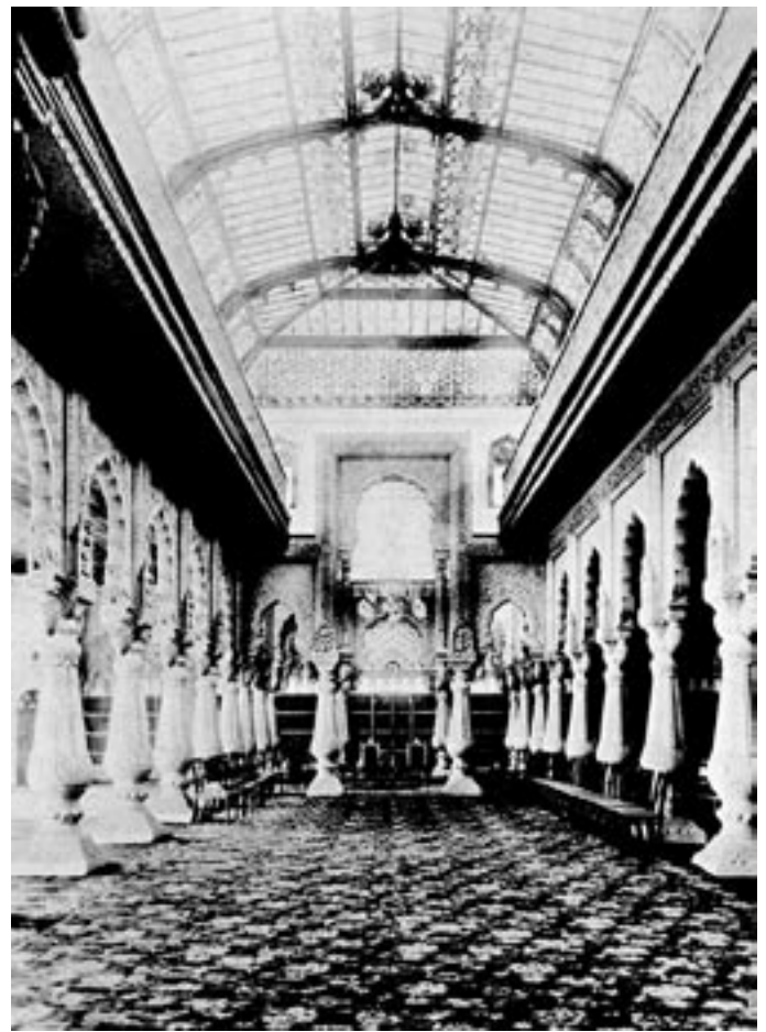
There was no architecture that could not be cast and moulded by McFarlane's of Glasgow in their black-sand iron-casting beds. This pre-fabricated Mogul-style Durbar Hall, was ready, in 1891, to be unbolted and shipped Empire-wards. Cast-iron Architecture was also a cast-iron investment. It could be unbolted and sold onwards, to a second site.
