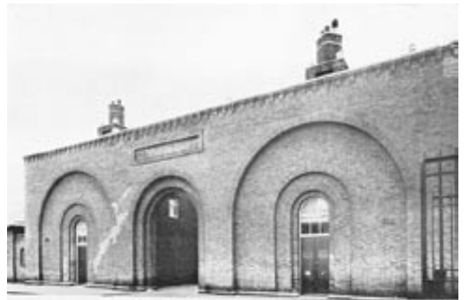
The 1814 Stables to the Royal Hospital at Chelsea manifest the wall as a unique succession of arched incisions worthy of an Egyptian 'door of appearances'. The entablature appears swallowed by the layers of wall in front of that the layer into which the doors are actually fixed.
